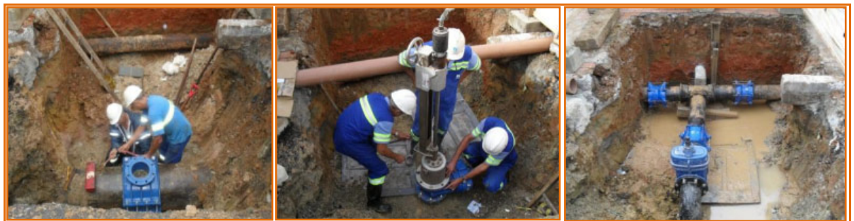
Figure 3 – Sequence of activities to interconnect a network in Alpina Village supply zone.
