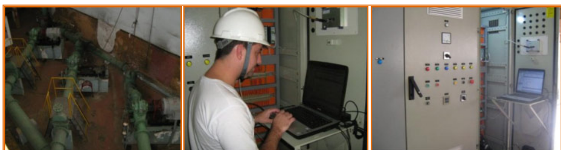
Figure 4 - water pumping station and the panel of the frequency inverter.
