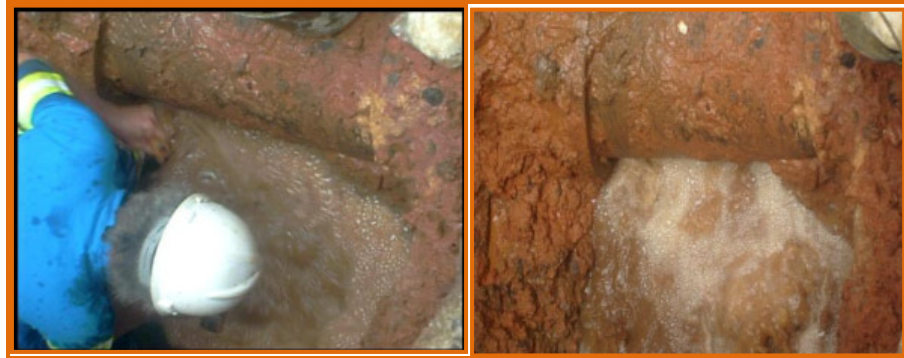
Figure 9 – Unreported leak located though PRV monitoring.
