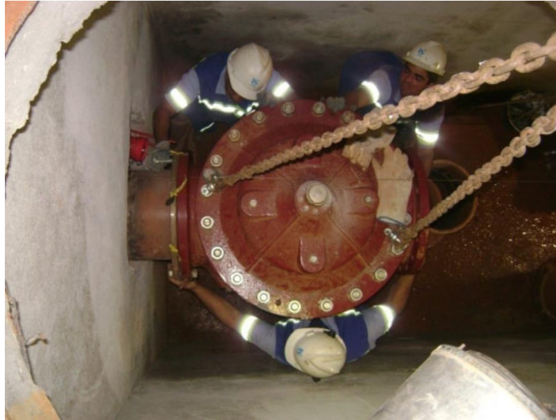
Figure 5 – Installation of a 400 mm PRV by Sabesp's labour (Source: Sabesp).
